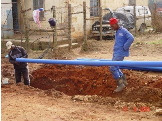
REPLACEMENT OF WATER PIPES IN UGIE, 2008
